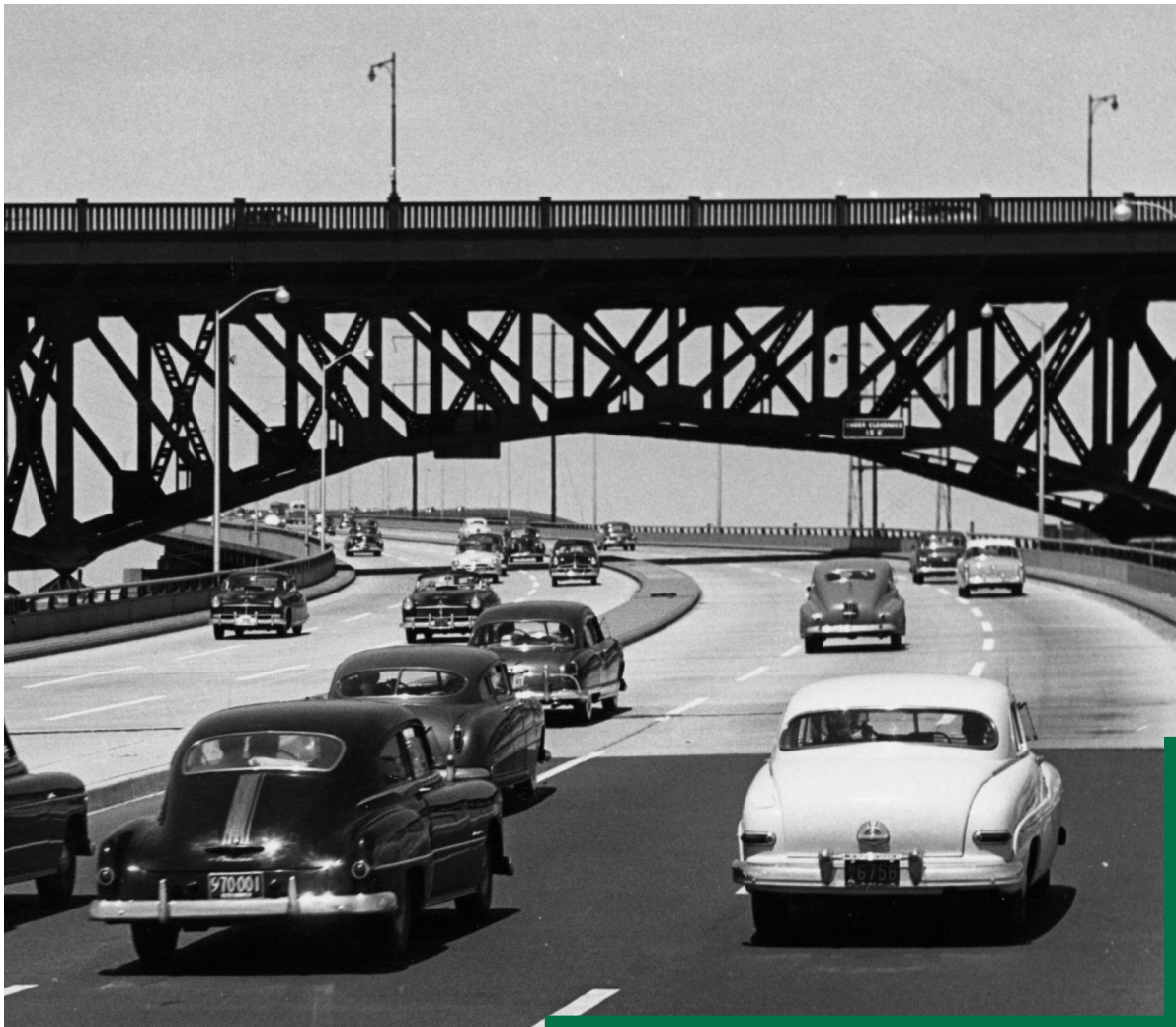
Under the Pulaski Bridge, New Jersey Turnpike - 1955
