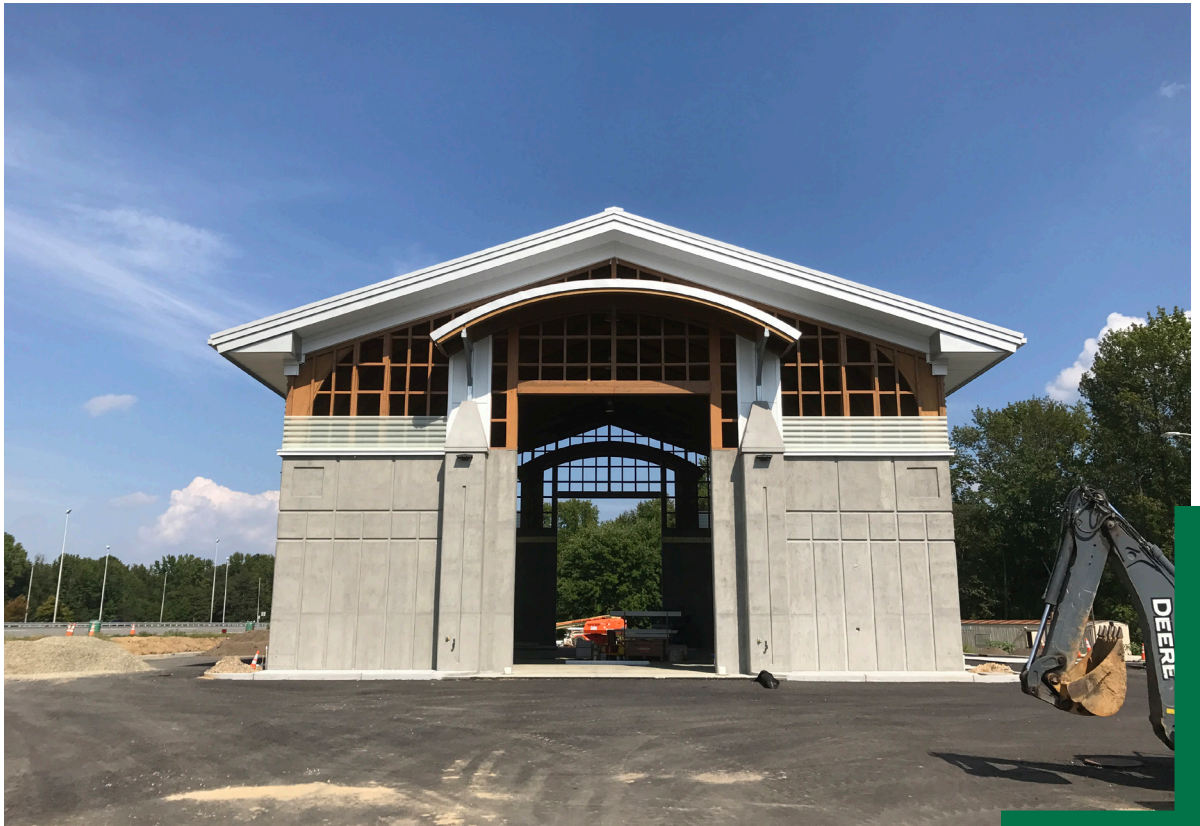
Salt Storage Facility, Interchange 1, New Jersey Turnpike - 2018
