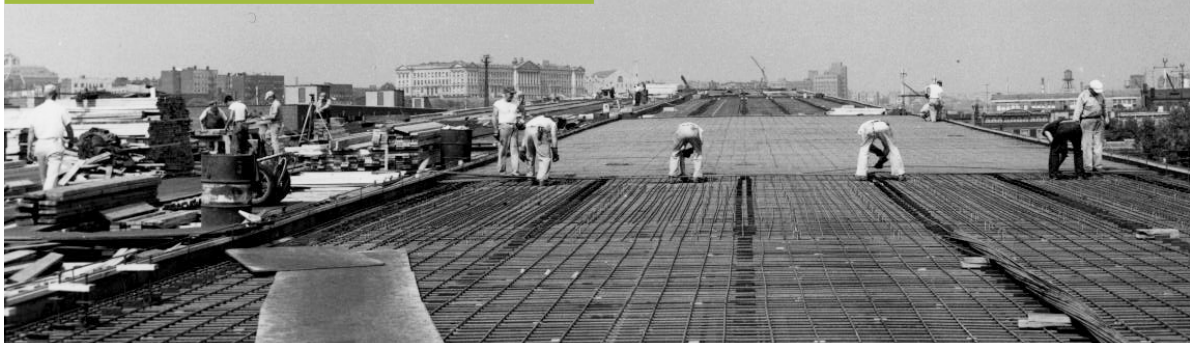
Newark-Hudson County Expansion, New Jersey Turnpike - 1955
